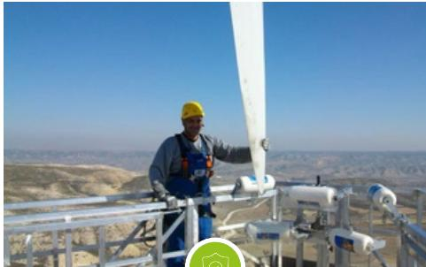
**PERMANENT PROTECTION ROLLER** In addition to four mobile rollers with K-BP-2L, we also provide extra permanently mounted rollers at the front side of the platform. It protects and guides, leading the edge of the blade smoothly.
